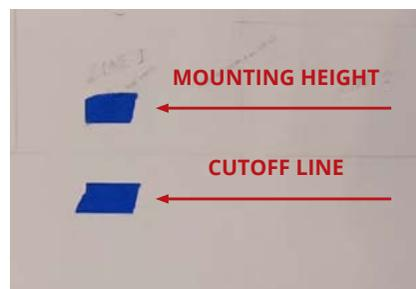
10. Mark the mounting height on the wall or garage door using tape.
